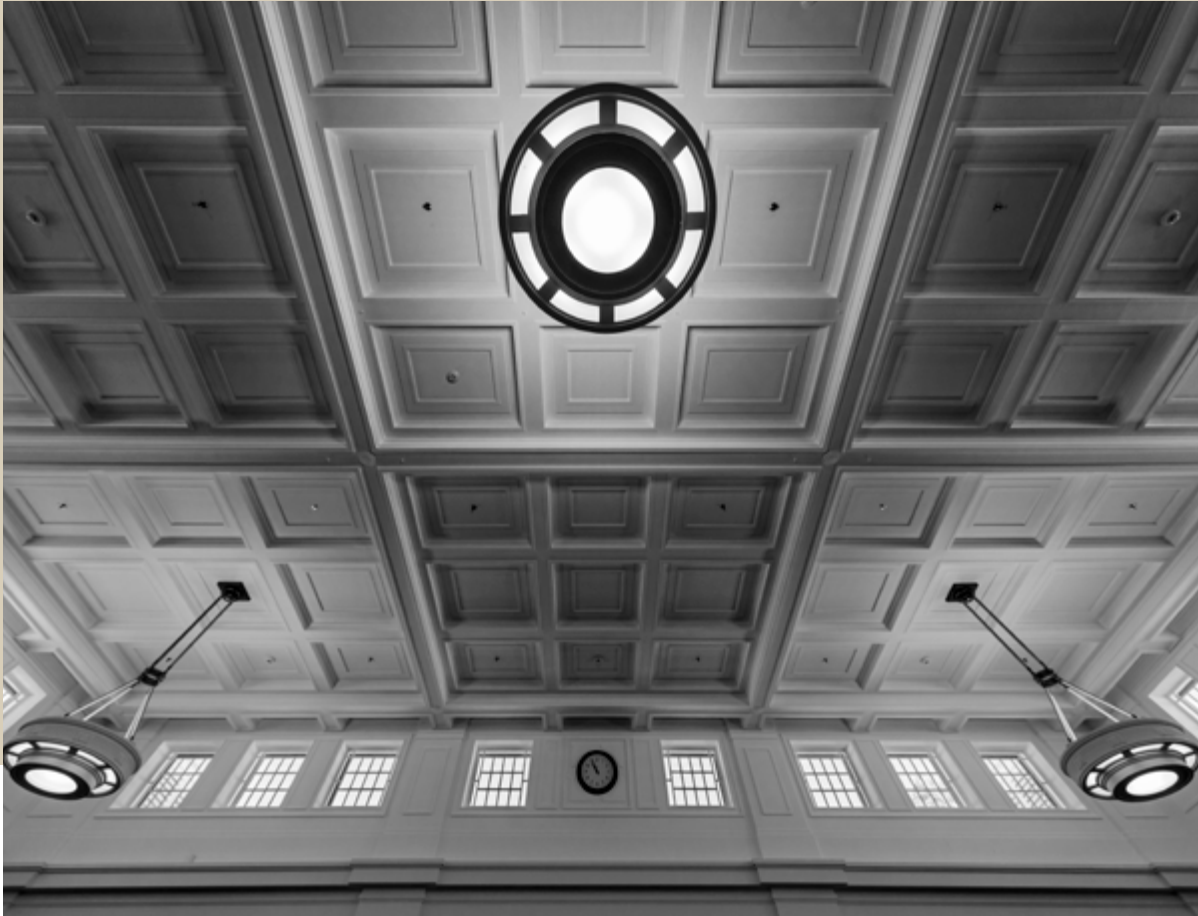
Ceiling detail from King's Hall Photo by: Andrew Merry
